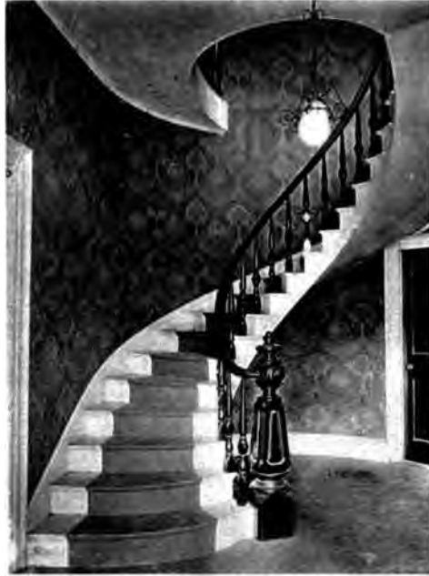
STAIRCASE IN HUNT HOUSE
